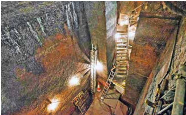
View from Level 3 at Paddington, looking down into Level 4. Photo Chris Rayner
